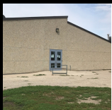
GRADE 5 SOUTHEAST DOORS
